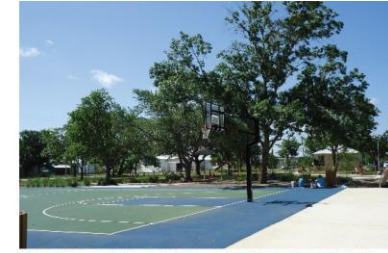
BASKETBALL COURT ENHANCEMENTS
