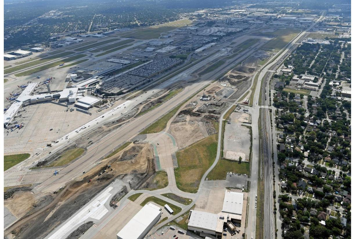
*Figure 2 - RWY 13R/31L and TWY C under construction*
