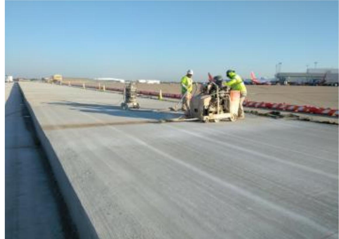
*Figure 6 - TWY C, final pavement layer installed, saw cutting underway*
