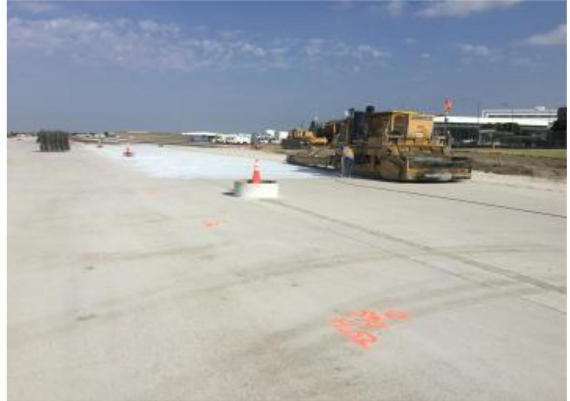
*Figure 4 - TWY C with sub layer installed, ready for final concrete layer*
