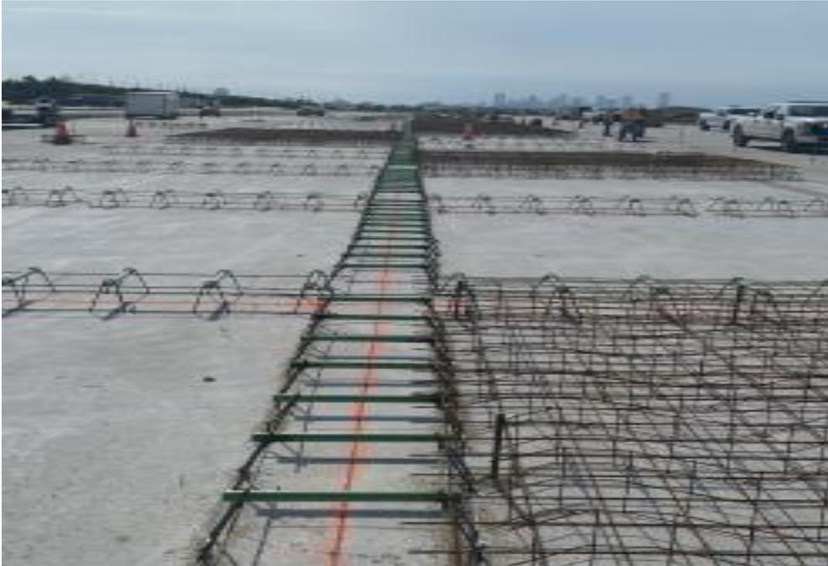
*Figure 5 - TWY C with reinforcements being placed in preparation for final pavement layer*
