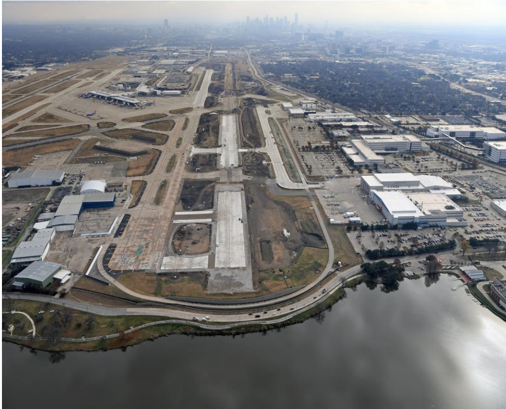
Figure 1 - RWY 13R looking SE
