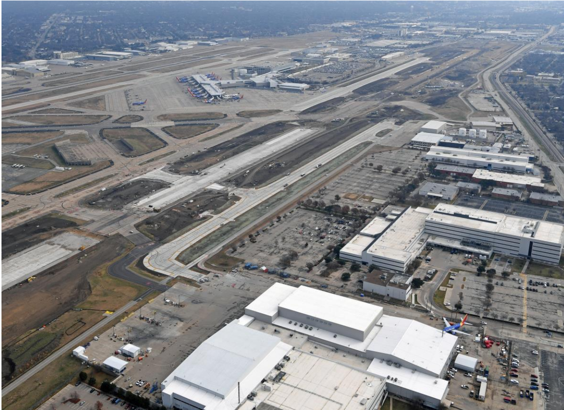
Figure 3 - New TWY T under construction (Phase 1) and north half of RWY 13R/31L under construction (Phase 2)
