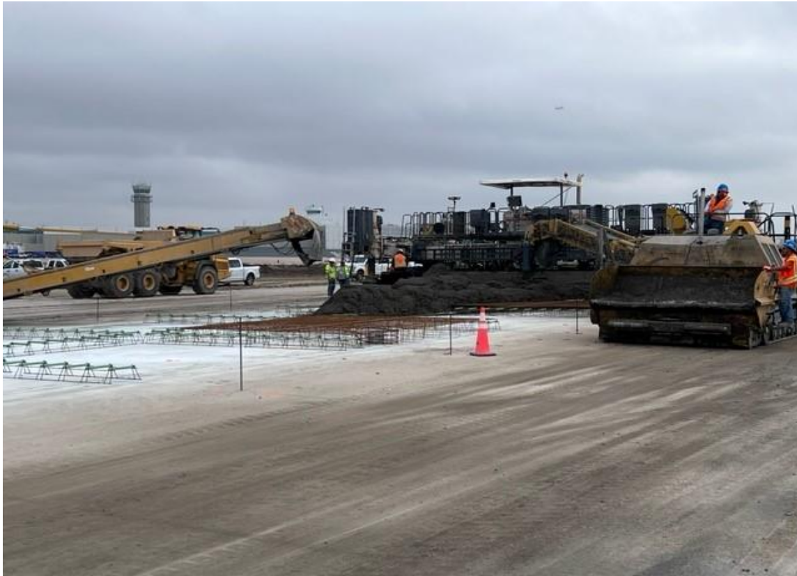
Figure 5 – RWY 13R/31L with reinforcements and placing final concrete pavement layer
