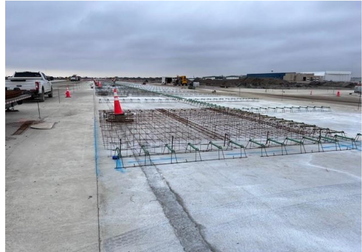
Figure 6 – RWY 13R/31L, final pavement layer preparation
