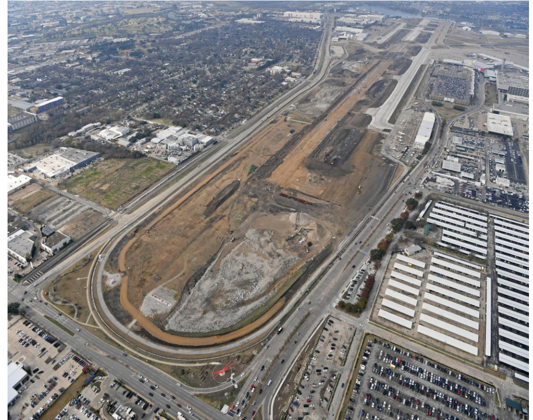
Figure 2 - RWY 13R/31L and TWY C under construction
