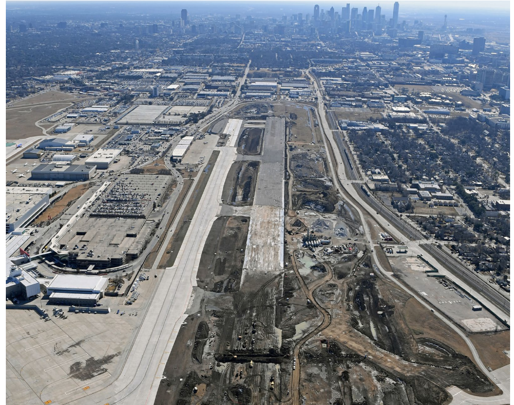
Figure 2 - RWY 13R/31L and TWY C NE
