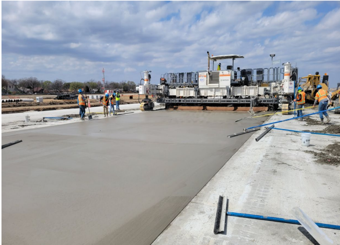
Figure 6 – RWY 13R/31L with reinforcements and placing final concrete pavement layer
