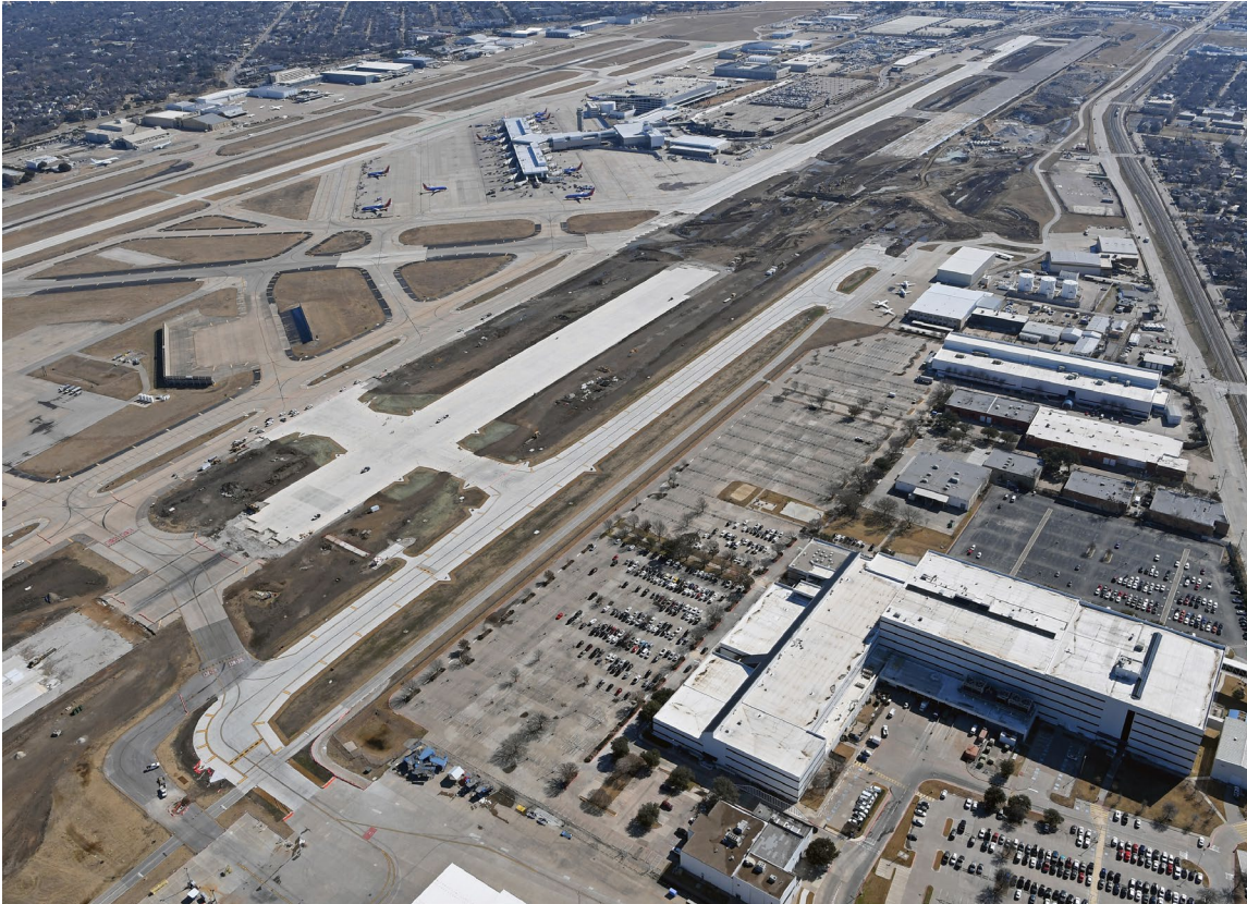
Figure 3 - New TWY T, TWY T 5, and TWY C 7 under operation
