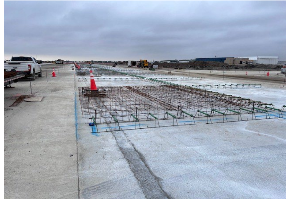
Figure 7 – RWY 13R/31L, final pavement layer preparation
