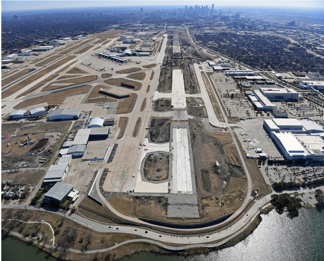
Figure 1 - RWY 13R looking SE
